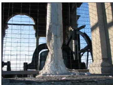
The 8 structural columns have to be replaced along with the balusters and rails.
